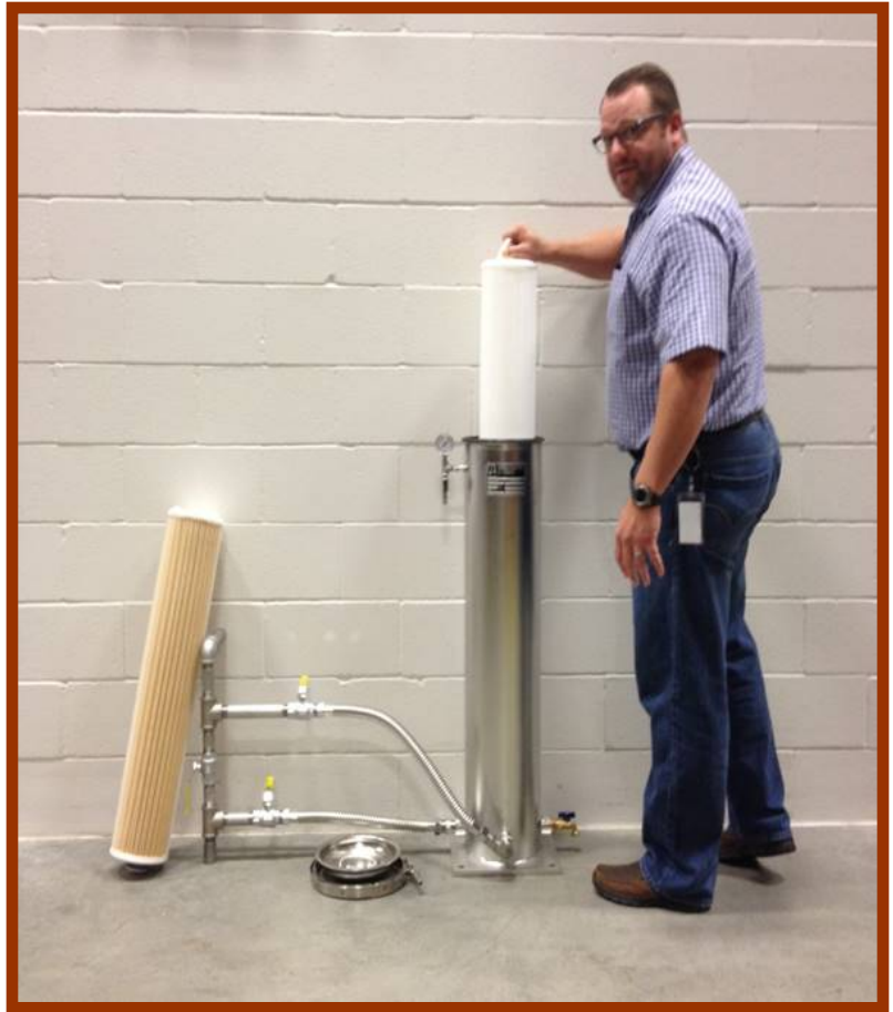
Vertical Filter Removal, Used Filter On Left, New Filter Being Installed
